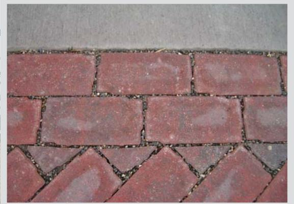
Aggregate sub base and base courses are used for pervious concrete and porous asphalt wearing courses. Permeable interlocking concrete paver installations require additional aggregate setting bed and joint fill.
