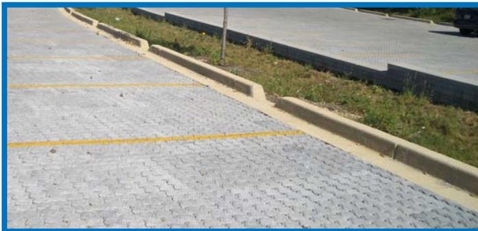
Multiple curb cuts allow flow into sumped landscaping without causing scour.
